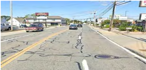
ADA compliance is thwarted in the Corridor, in part, by utility poles and discontinuous, substandard sidewalks.
