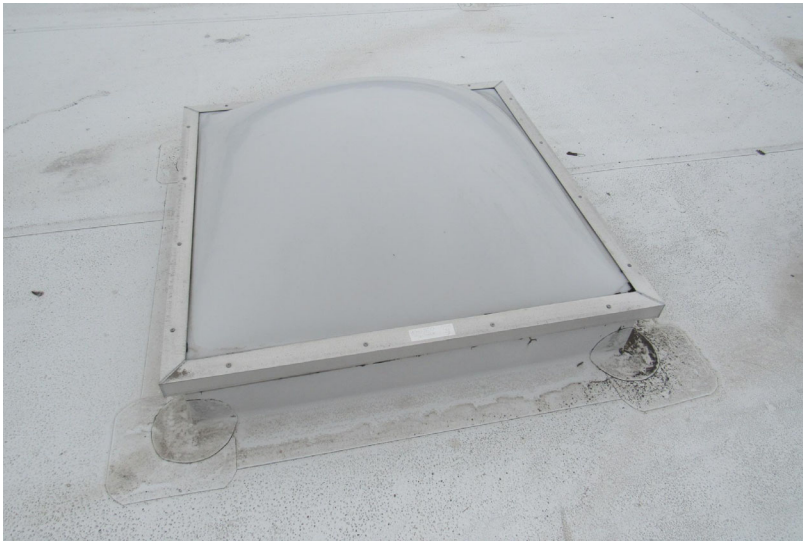
View of typical curb-mounted skylight conditions
