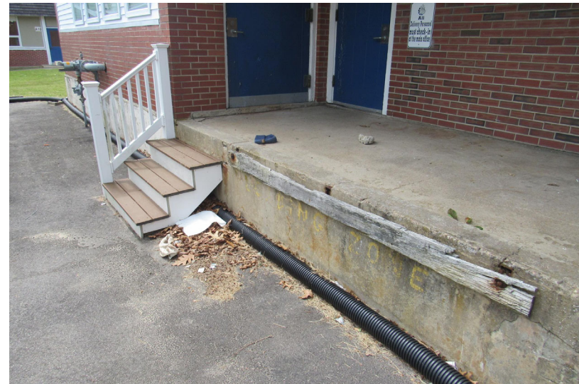
View of concrete loading dock present at north end of building
