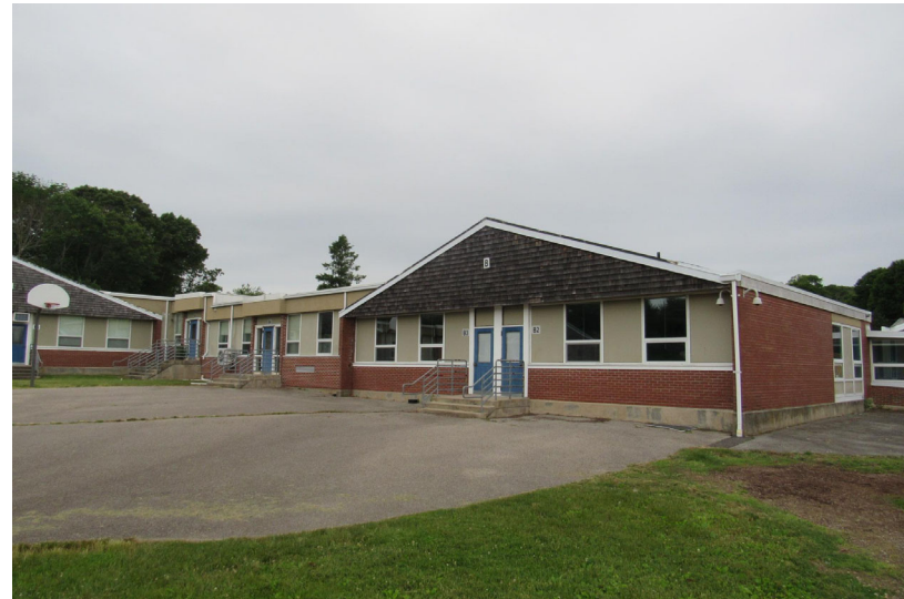
View of building architecture as seen at rear of building
