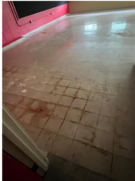
Figure 21: Asbestos floor tiles
