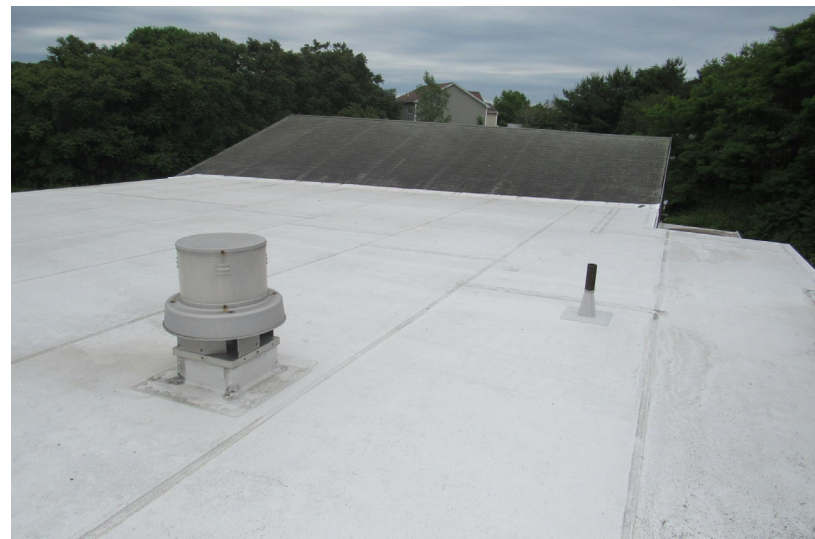
View of single-ply thermoplastic polyolefin (TPO) roof assembly conditions
