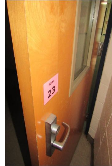
View of typical interior passage doorway conditions
