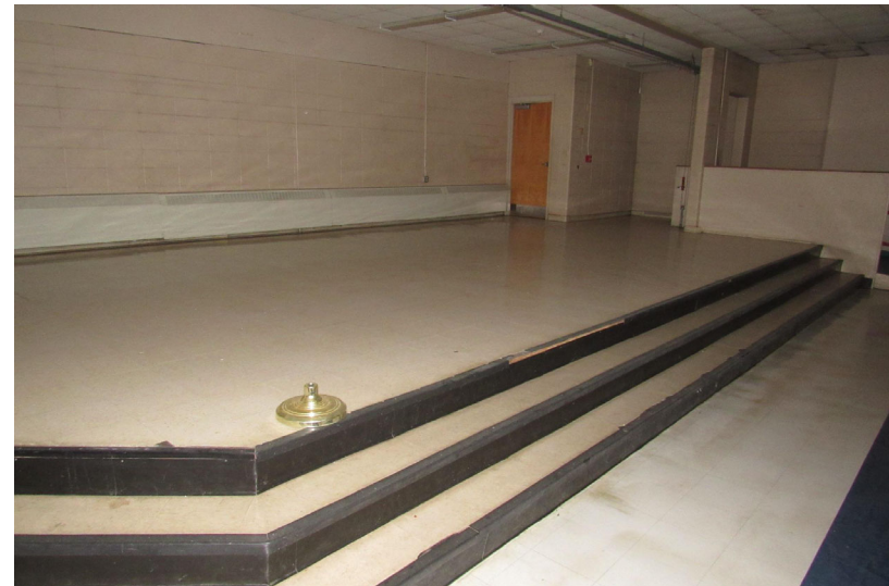
View of auditorium stage finishes
