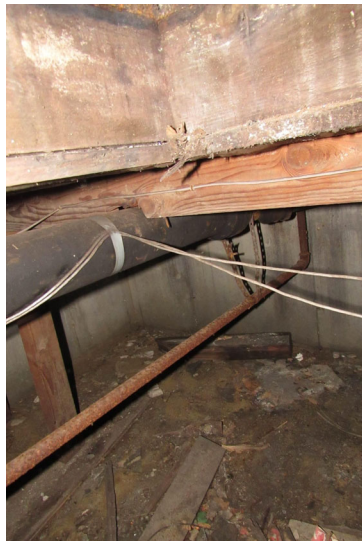
View of sample of building crawlspace conditions
