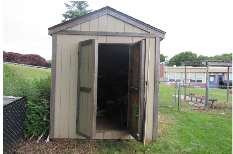
View of rear wood-framed storage shed
