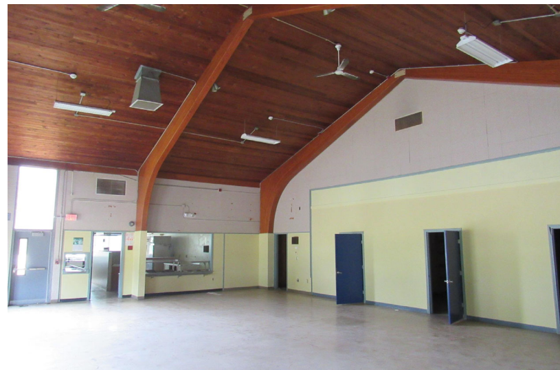
View of cafeteria finishes – commercial kitchen in background
