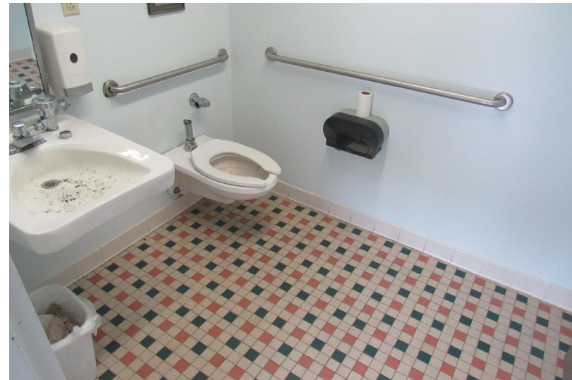
Additional view of common restroom finishes and fixtures
