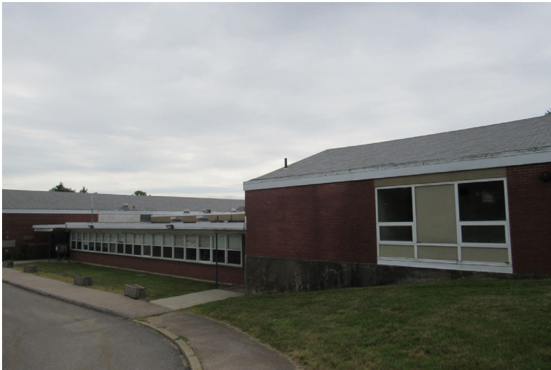
View of building architecture as seen at front of building
