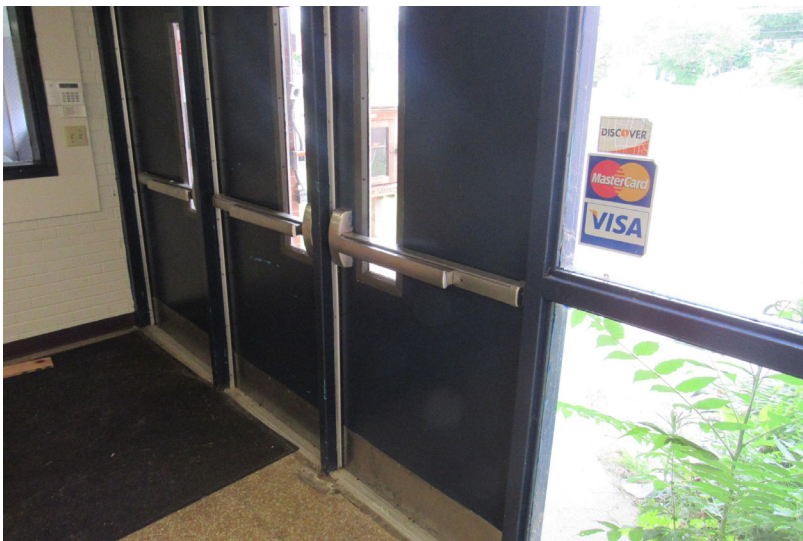
View of main entry metal doors with vision panels
