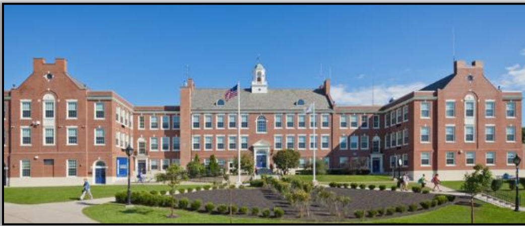
Figure 3-5 Westerly High School (Photo Credit: Mary Adams)
