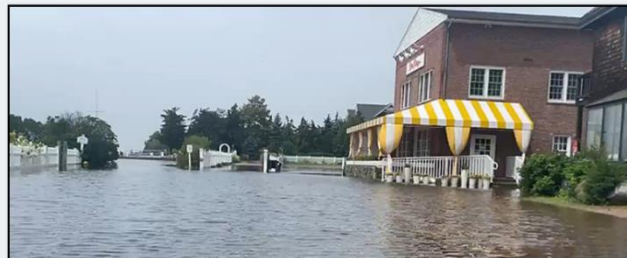
Flooding from Tropical Storm Henri Watch Hill Court August 22, 2021 Photo Credit: WJAR/turto10.com
