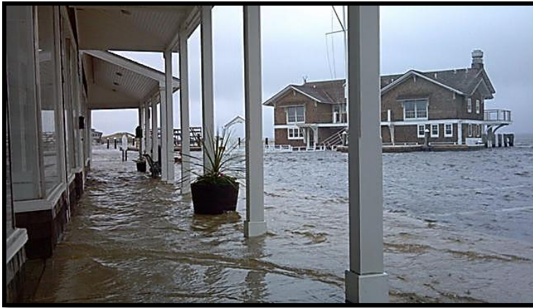
Figure 4-14 Storm Surge Flooding from Superstorm Sandy (October 2012)
